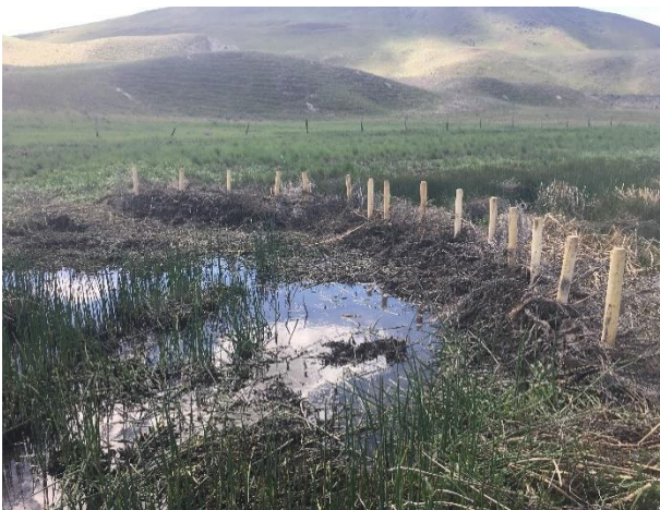
Figure 11: BDA on the Day of Installation in Spring PC: Foster Creek Conservation District
