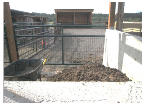
After photo of Heavy Use Area and waste storage.
