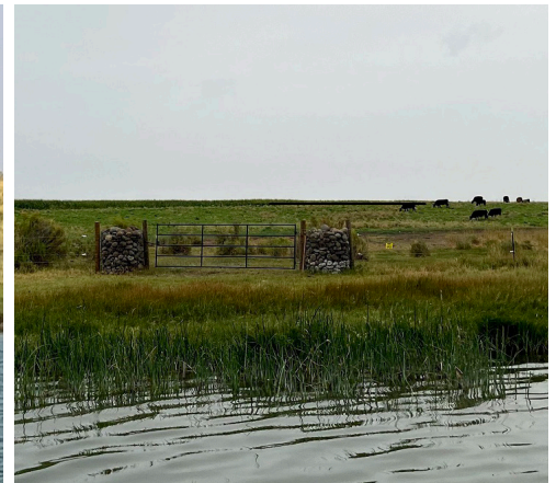
Left: Before Project - Uncontrolled access to shoreline. Design and layout completed, cultural resources investigation pending. (photo by Lyle Stoltman) Right: Completed Project - Livestock exclusion, rock cribs, 4-strand electric fence and gate for maintenance and landowner access. (photo by Kristina Ribellia)
