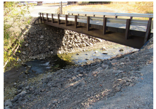
Site before the project started (top) and after it was complete (bottom). (photos by Dave Hedrick)
