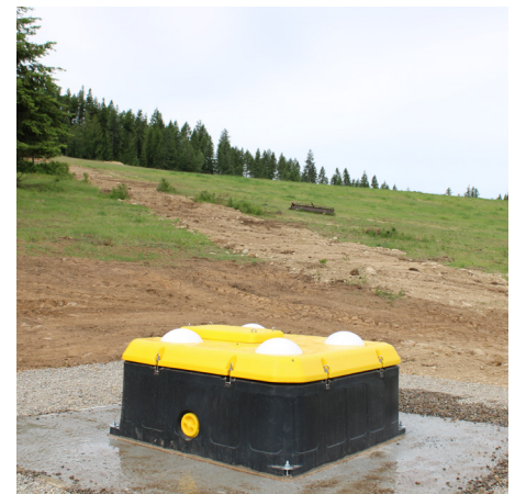
Completed project showing frost-free water tank, length of livestock pipeline, and slope from pre-drilled well. (photo by Mary Malone)
