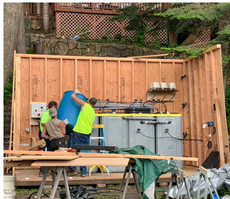
Photo of the Busse system being installed.
