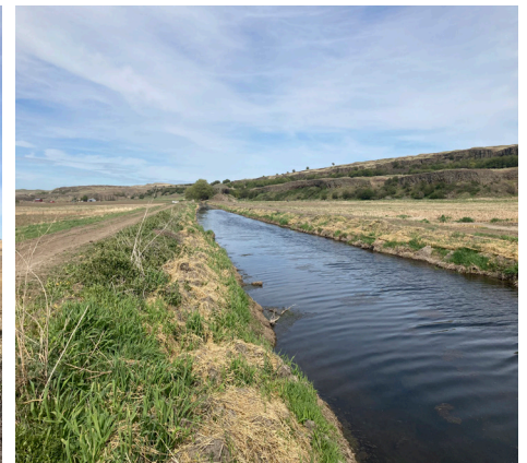
Kamiache Creek functions again as a stream, meanwhile new grasses grow on the banks.
