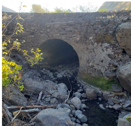
Left: Before construction - corrugated round culvert created barrier for fish passage. Right: After construction - three-side concrete box culvert allows fish passage at all flow levels.
