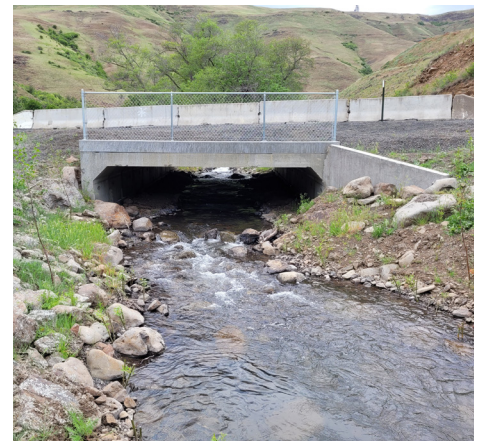
Left: Before construction - corrugated round culvert created barrier for fish passage. Right: After construction - three-side concrete box culvert allows fish passage at all flow levels.
