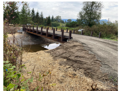
A new bridge over Haystack Creek opens the stream channel for fish and reduces the risk of flooding the private road. (photo by Snohomish Conservation District)
