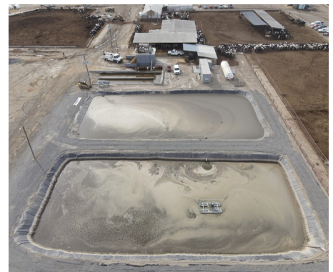
Dairy waste separation facility (looking south) containment runoff control structures. Photo by landowner.
