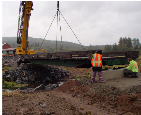
Left: Construction team placing bridge over Gosnell Creek to eliminate a wet crossing and improve in-stream conditions. Right: Restoration crew members, Marissa Newby and Justin Leigh installing exclusion fencing along Gosnell Creek. (photos by Mason Conservation District)
