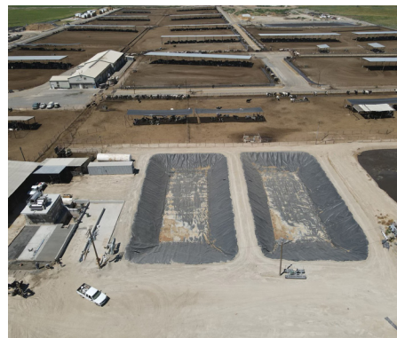
Dairy waste separation facility (looking west). Screened solids slab, sand lanes and two synthetically lined settling basins. Photo by landowner.
